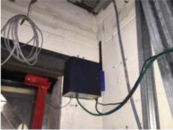
*IC Sentinel® monitor placed inside a construction Anteroom, with differential pressure probe and Cellular Data Modem*
