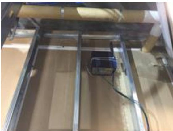
*IC Sentinel® monitor placed inside a construction barrier, with differential pressure probe and Cellular Data Modem*
